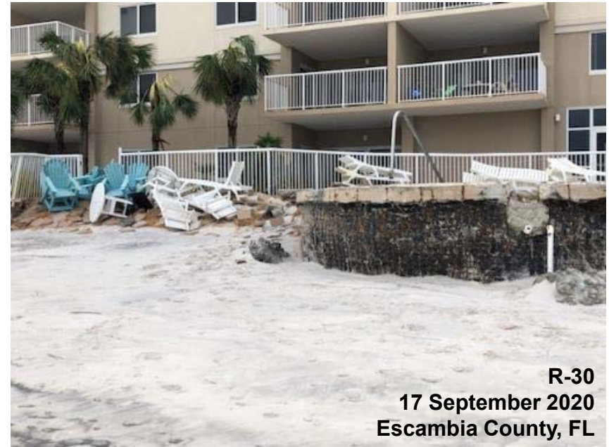
R-30 17 September 2020 Escambia County, FL
